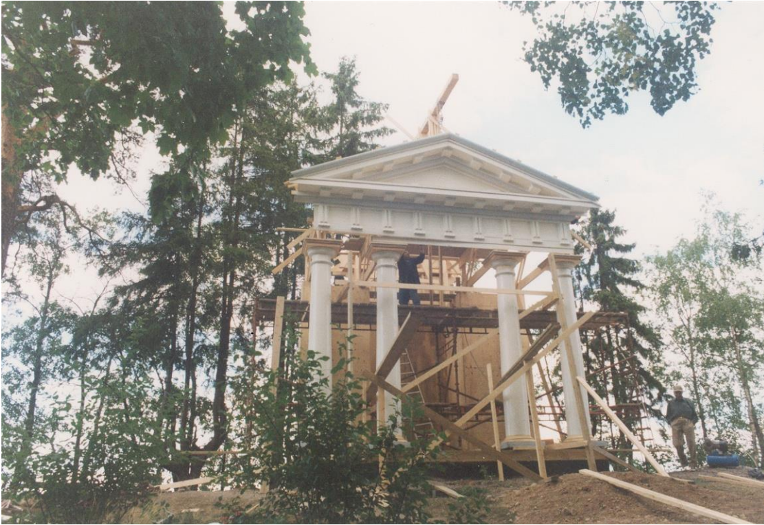
Picture 85. The cornice panel is being hoisted. (TAMK)
