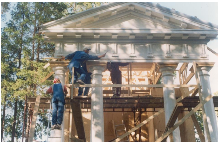
Picture 89. The cornice panel is attached. (TAMK)
