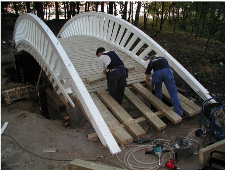
Picture 138. Installing the deck of the bridge. (TAMK)
