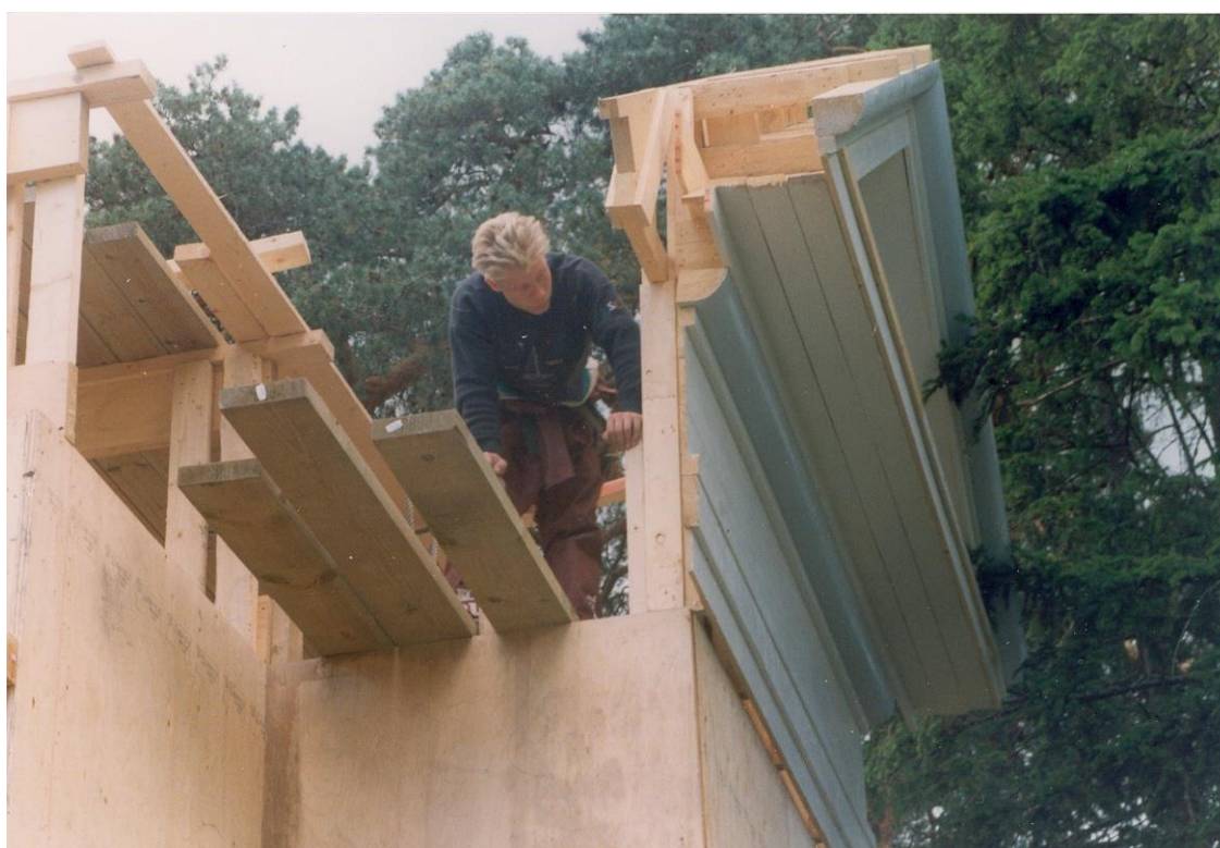
Picture 84. Joni Virtanen attaching an eave. (TAMK)
