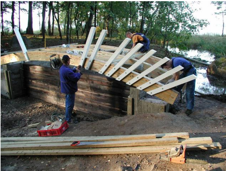
Picture 135. The prefabricated studs had to be carefully put to place. (TAMK)
