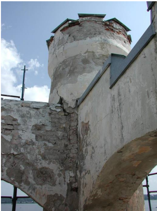
Picture 117. Cracks between the towers. (TAMK)
