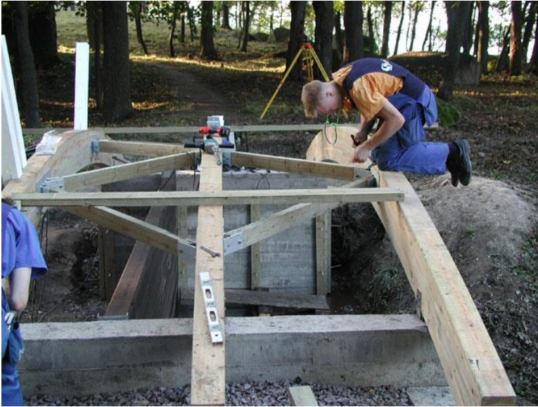
Picture 134. The beams were supported to prevent fluctuation. (TAMK)
