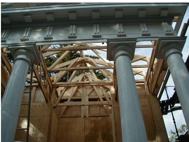
Picture 92. Mr Koreasalo's ingenious design for the roof: The roof is supported by struttet trusses leading from the pillars to the back wall. On top of these laminated girders will be placed.
