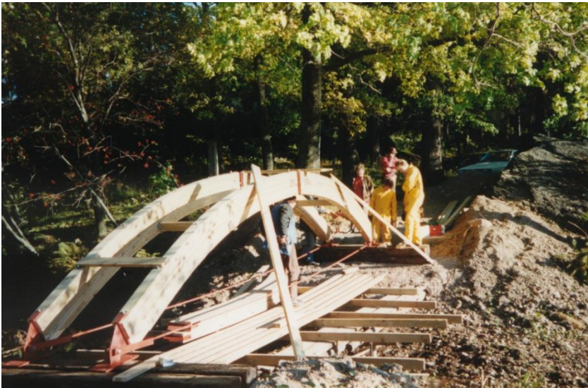
Picture 59. Arched beams being made. (TAMK)
