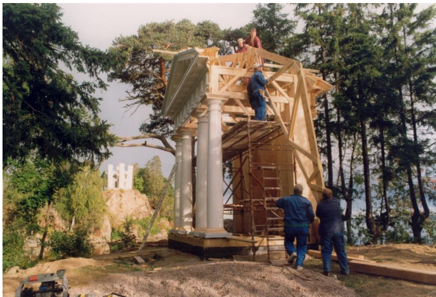
Picture 87. The roof truss is being lifted to its final position. (TAMK)
