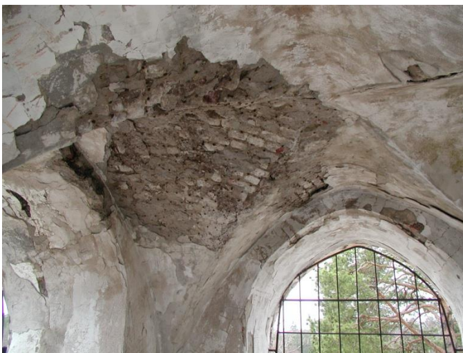
Picture 118. The plastering in the vaults is coming off. (TAMK)
