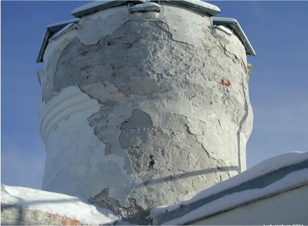
Picture 121. The result of the plastering carried out in December 2003! Picture from 2004. (JL)
