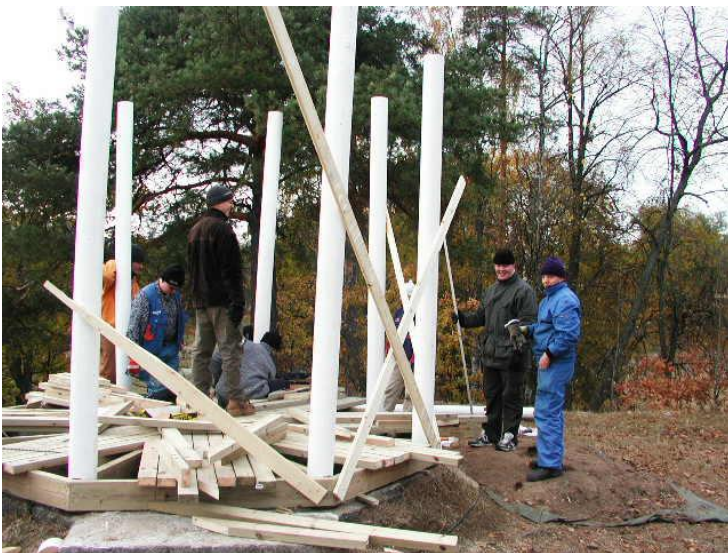
Picture 157. The ready painted poles are erected. (TAMK)
