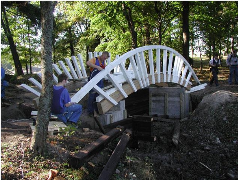
Picture 137. Preparations for the handrail to be installed. (TAMK)
