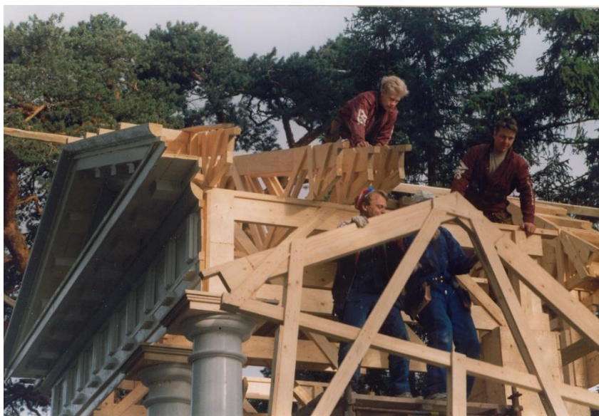
Picture 88. The truss for the back follows. (TAMK)
