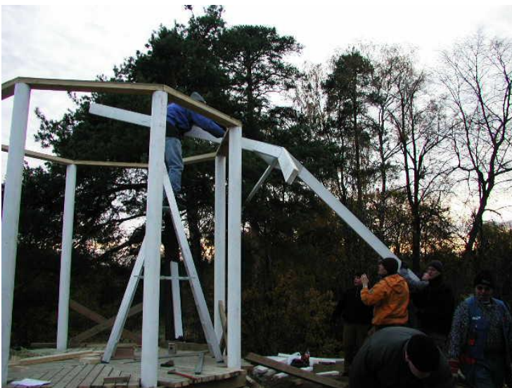
Picture 158. The supporting beams for the roof are erected. (TAMK)
