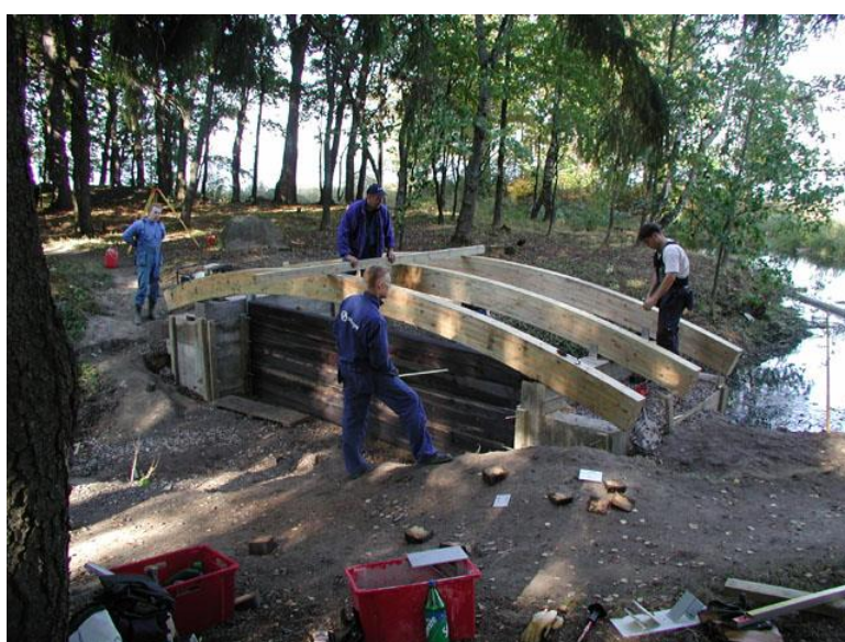
Picture 133. Final measuring and adjusting the beams. (TAMK)
