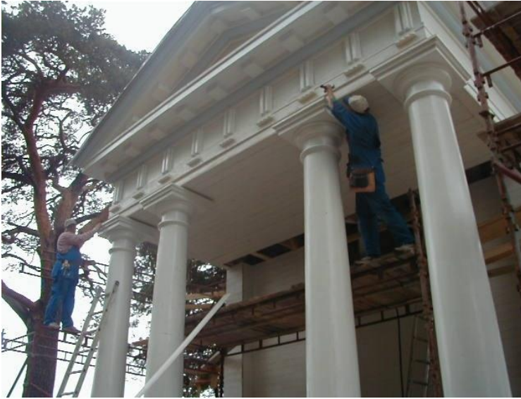
Picture 96. Final touches. The pillars taper upwards. (TAMK)
