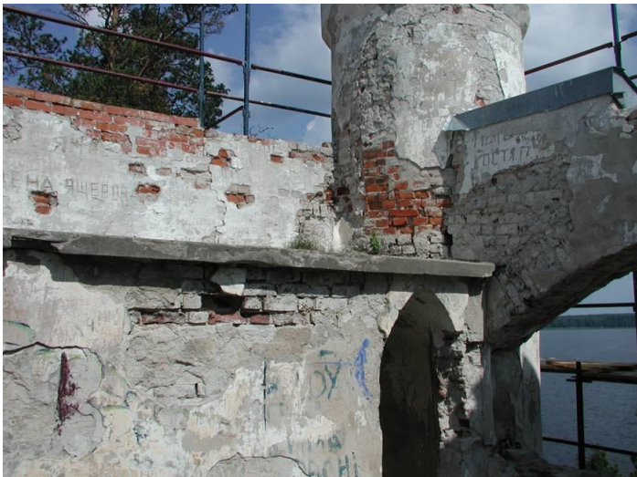
Picture 115. Plastering has come of taking some of the tiling with it. (TAMK)
